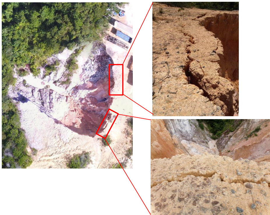
Figure 14. Rills along the margin of Gully 01, Distrito Industrial II neighborhood. Source and prepared by the authors (2026).
