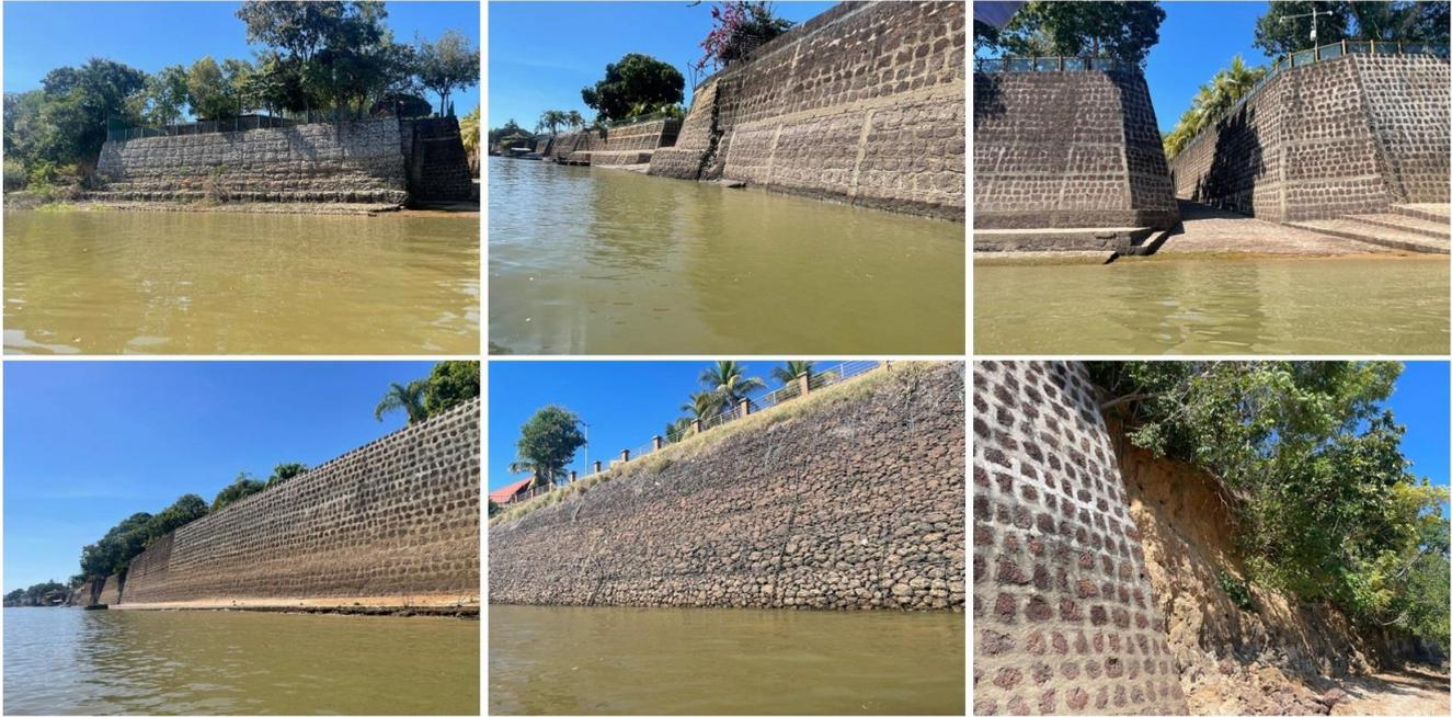
**Figure 14.** Containment structures at the Araguaia and Vermelho River confluence, from the right bank of the Vermelho River to downstream of the confluence. Source: The authors, 2025.
