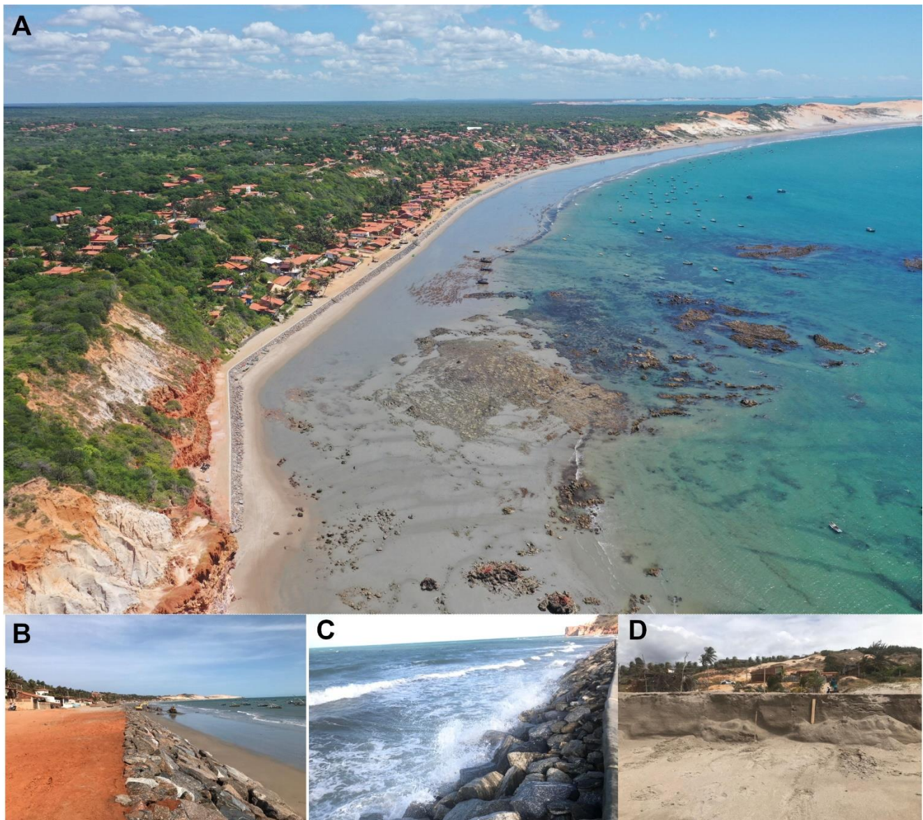
Figure 15. Mosaic of images: (A) West view of Redonda beach, showing a rock-fill coastal protection structure, which fixes the coastline; (B) Conclusion phase of the coastal protection work; (C) Incidence of waves on the protection structure; and (D) An erosive scarp more than half a meter high.
