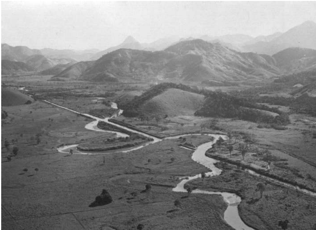
Figure 4 - A channelized section of meandering sand bed river along the lower course of the Macaé River. This photograph picture was part of the collection from the now defunct agency DNOS (National Department of Construction and Sanitation; now part of the Municipal Public Archive Waldir Pinto de Carvalho (Campos dos Goytacazes, RJ).
